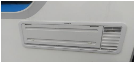
Photo 33. Ventilation grille outside the caravan
