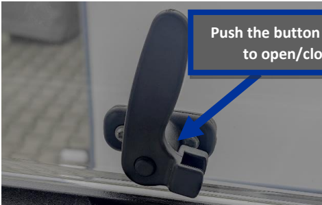
Photo 12. Window handle unlocked
