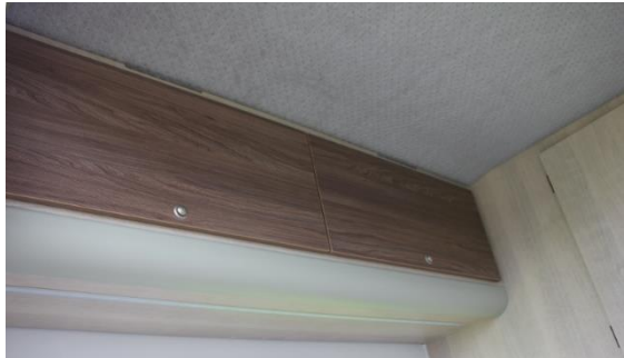
Photo 38. LED strip under the cabinet above the hob
